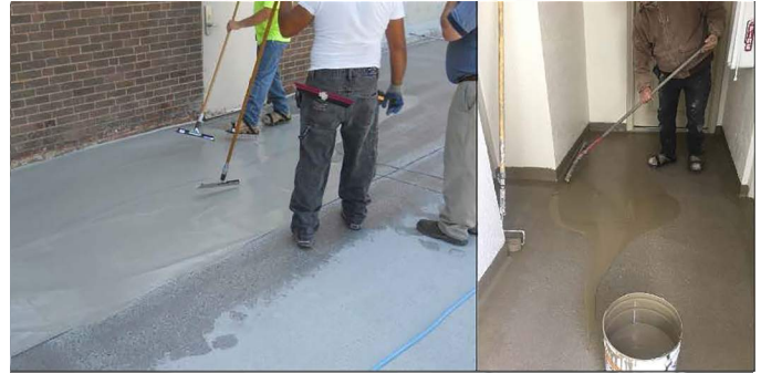
Fig. 7: (a) Cementitious and (b) polyurethane deck coatings
