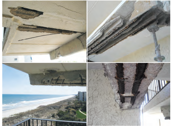
Fig. 2: Corrosion damage: prestressed hollow core panels at Level 1 walkway soffit (top left), balcony prestressed hollow core panel during construction demolition (top right), balcony cantilever beam (bottom left), and walkway beam (bottom right)
