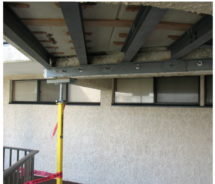
Fig. 3: Example of supplemental supports prior to project to make conditions temporarily safe
