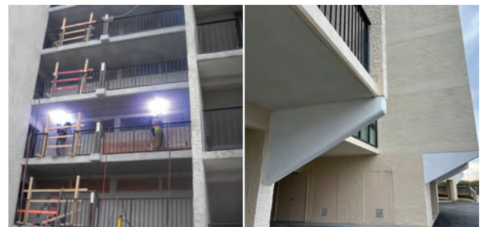
Fig. 10: Thermal spray being applied to the PHCP soffits (left) and current condition of haunches after thermal spray and coating application (right)
