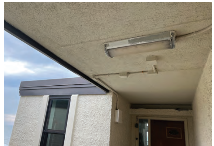
Fig. 11: Test station for CP testing at panel
